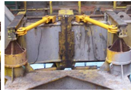
Added New Bracing
