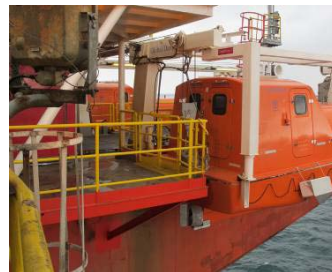
AFT lifeboat platform deformation
