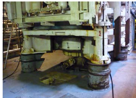
Existing Spider Frame with Wellhead Connector
